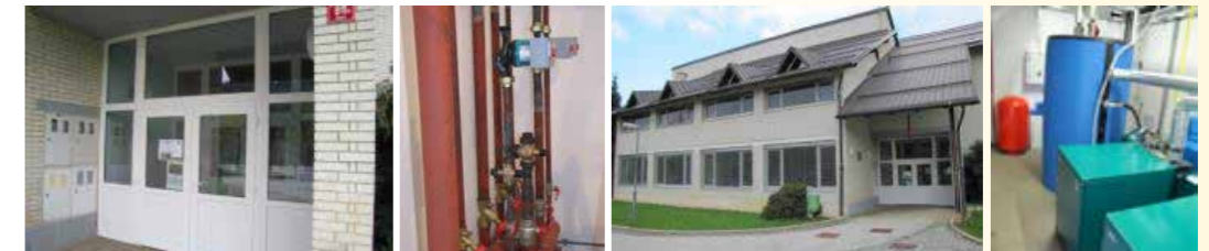
Figure 11: CHP POŠ Škale
