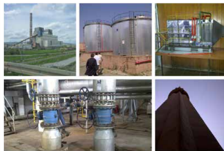
Figure 8: CHP plant in Pristina
